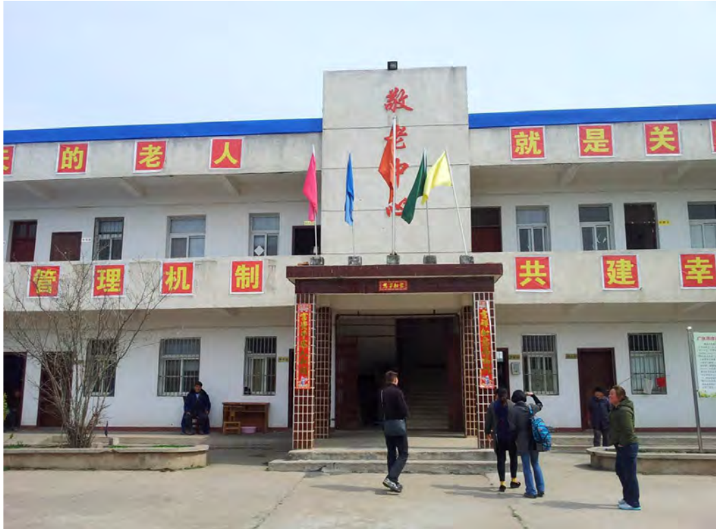
Former school in Hubei Province, converted into a home for the aged. Photo: Misereor.
